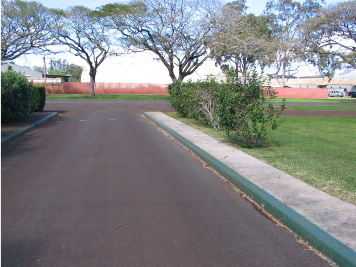
Figure 22: The Entry Driveway into the Post Cemetery
